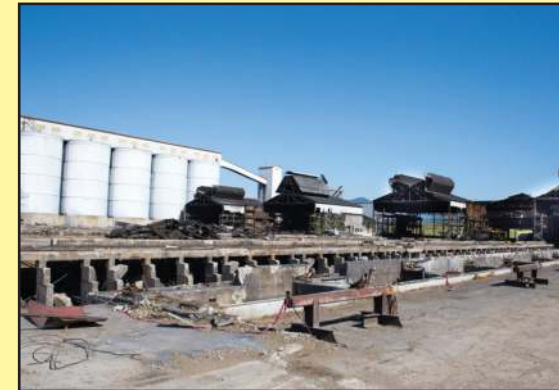
Last remnants of potrooms at the site.
