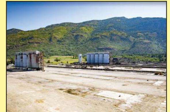
Backfilled potrooms 1-3 basements. The ore silos are to be demolished next.
