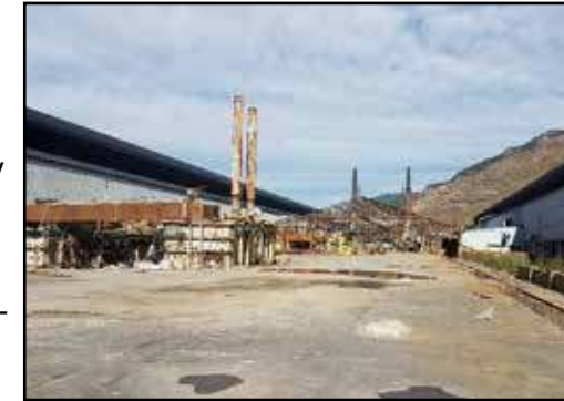
Former casthouse removed
