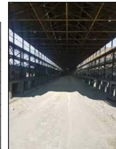
Potroom 2 with anode, cathode and basement concrete removed
