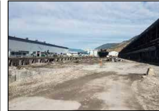
Potroom 1 structure removed
