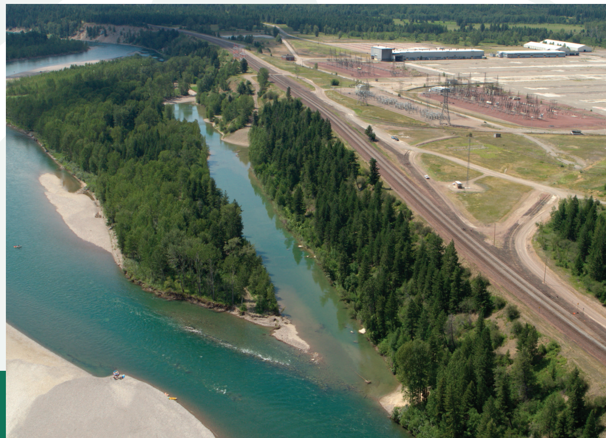
Flathead River and former South Ponds area (looking west), Summer 2021.
