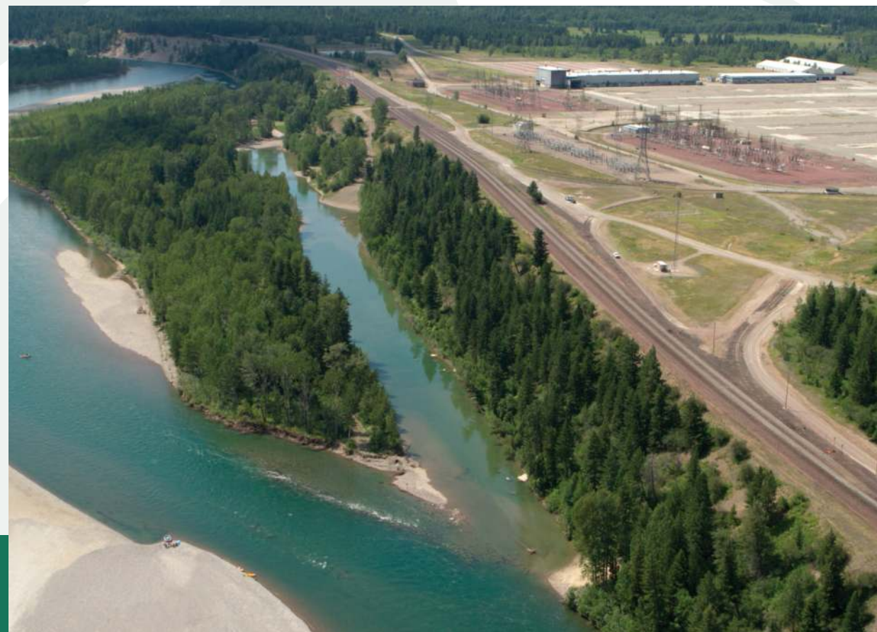
Flathead River and former South Ponds area (looking west), Summer 2021.
