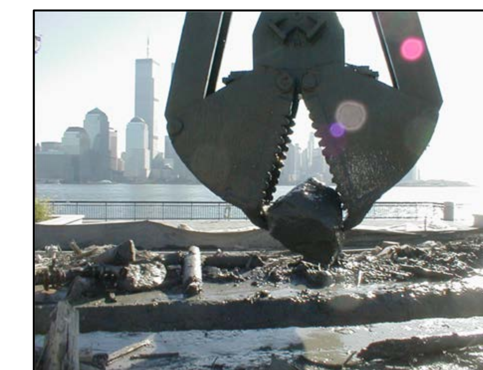
±2 ft boulder removed with clamshell bucket
