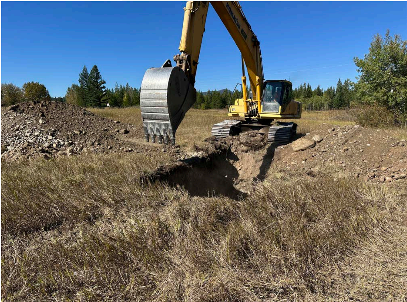
Equipment used for conducting the geotechnical investigation test pits adjacent to the west landfill.
